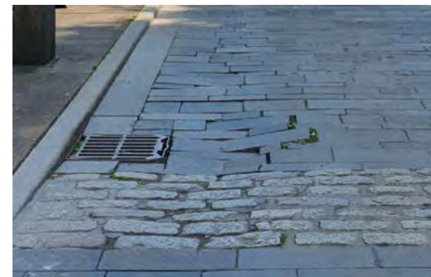
9.19 Castle Street surfacing
