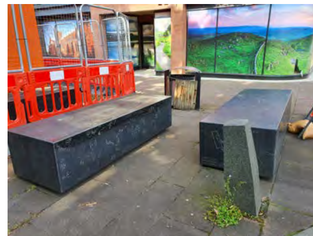
9.18 Castle Street failing and poorly maintained public realm furniture
