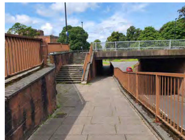
9.15 Underpass below Castle Way
