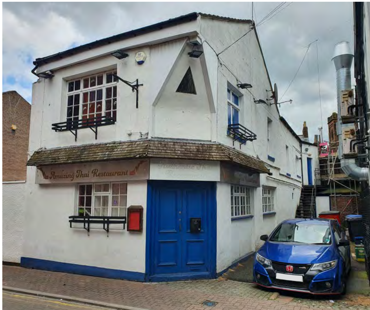
9.6 Inappropriate alteration has taken place to this historic building on Crosby Street
