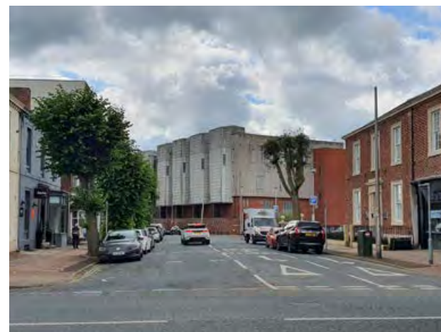
9.3 Adverse impact of scale, massing and design of the telephone exchange, Cecil Street
