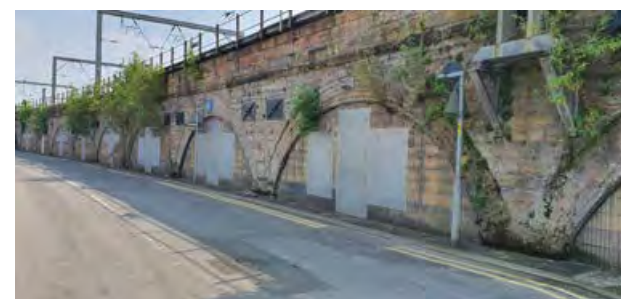
9.9 Vacant arches beneath the railway have significant potential as part of regeneration plans
