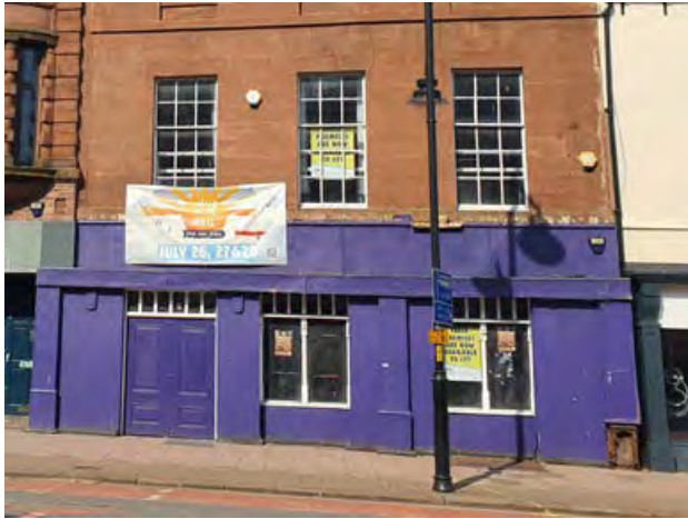
9.11b Poorly maintained retail unit in an inappropriate colour
