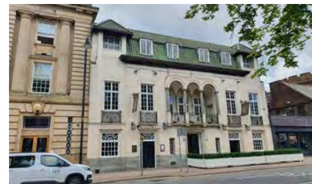
5.24 The Andalusian, Warwick Road, originally the Crescent Inn, and a Board Public House.
