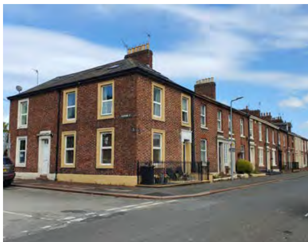
5.38 Terraces on Corporation Road
