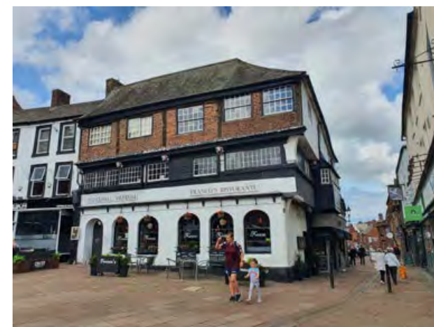
5.10 The Guildhall remains possibly the last timber framed building in Carlisle
