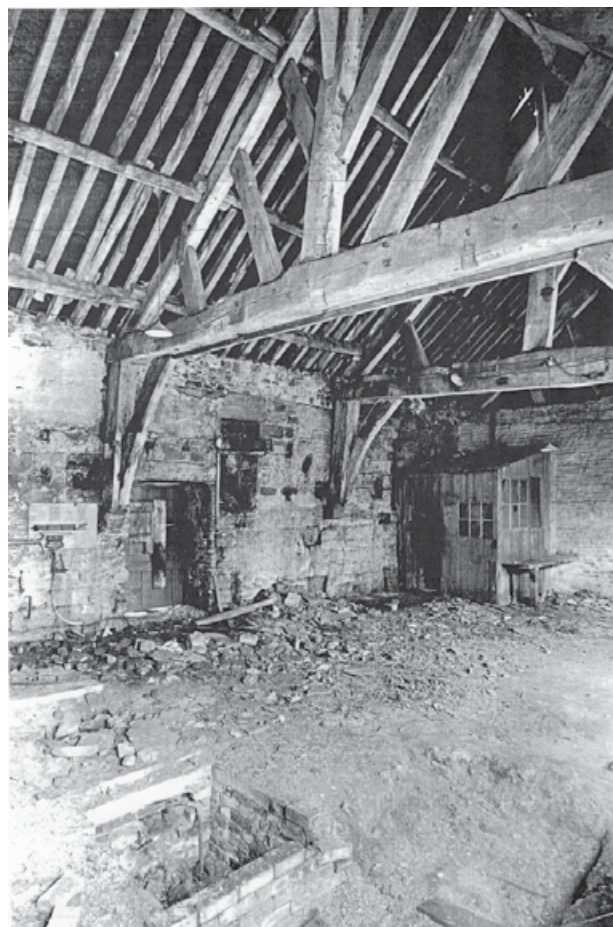
3.38 The Tithe barn interior before restoration (Carlisle Civic Trust)
