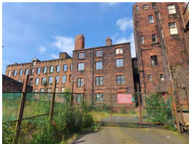
5.17 Warehouses from English Damside
