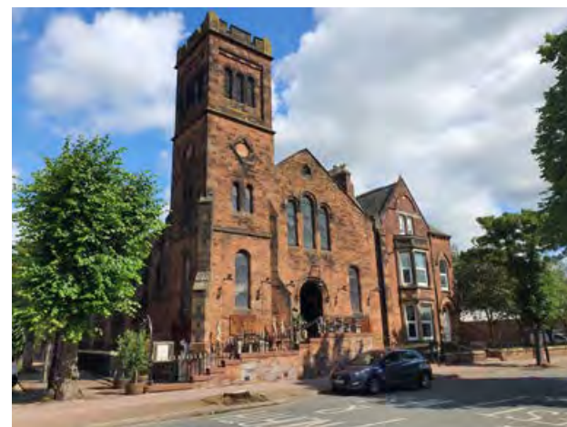
5.7 Former Warwick Road Presbyterian Church, now a restaurant
