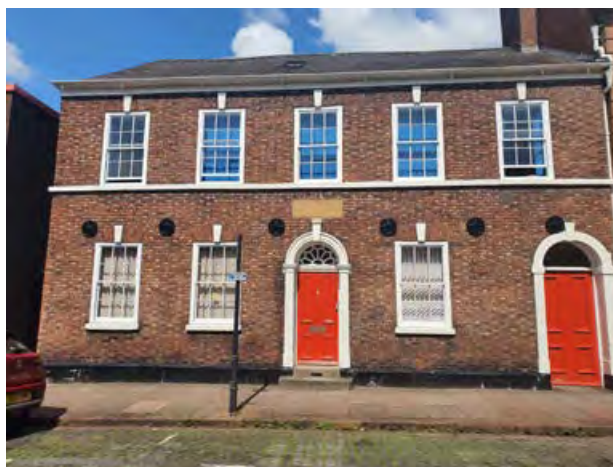
5.34 Late 18 th century house in Abbey Street
