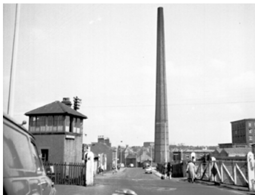
3.31 Shaddon Mill Chimney seen in 1966 from Dalston Road
