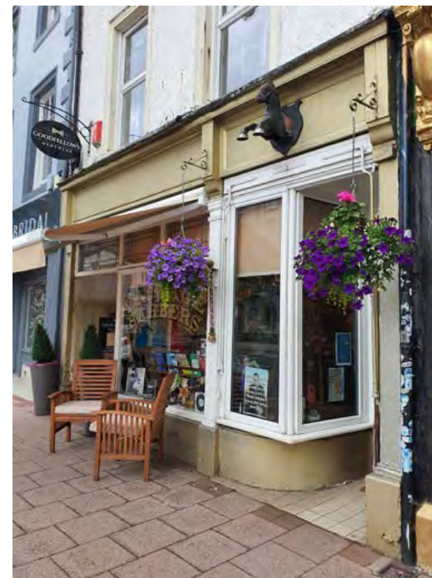
5.30 Historic shop front on Warwick Road
