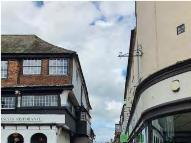
Panoramic views from the Irish Gate Footbridge towards the Cathedral along Abbey Street
