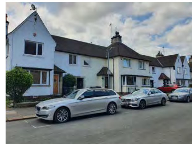
5.39 1930s housing, Warwick Street
