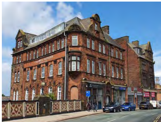
5.16 Solid Victoria commercial with elements of Classical Flemish Revival style
