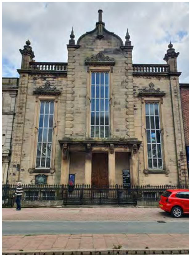
5.5 Carlisle City Church
