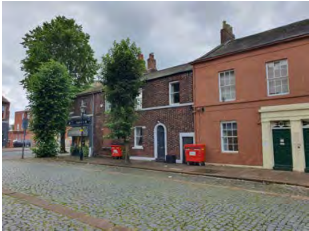
Former town houses on Earl Street
