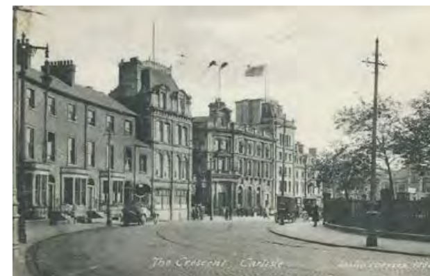
7.11 The Crescent, looking towards the railway station, before the shopfronts were added (Cumbria Image Bank)
