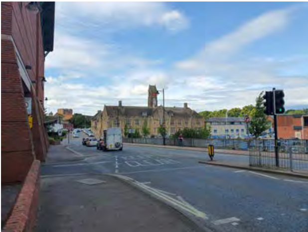
The tower of the Old Fire Station seen from West Tower Street and falling topography
