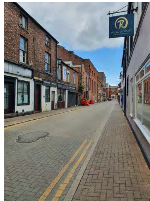
Crosby Street retains a number of its historic warehouses and workshops
