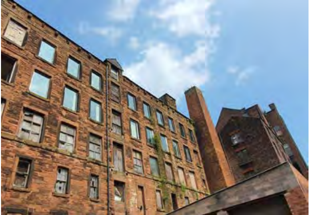
Former warehouses from English Damside
