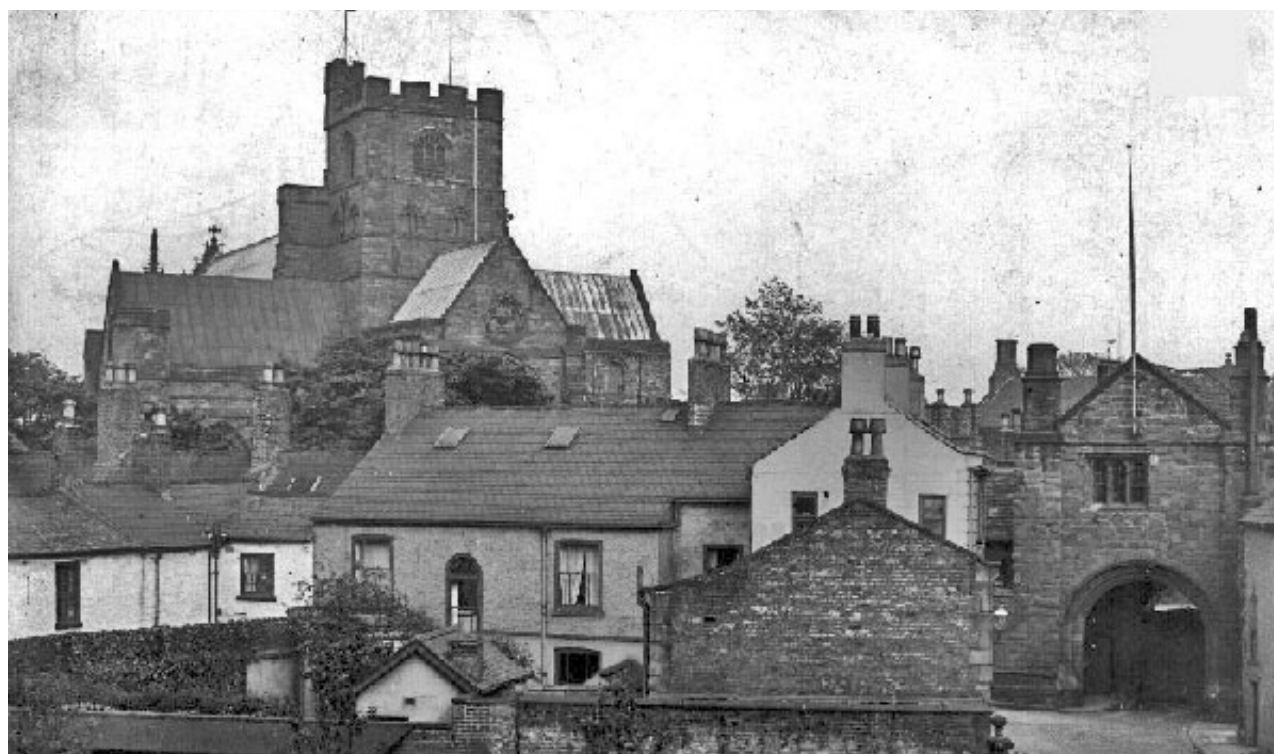
7.5 The Cathedral and Precinct from Abbey Street c1900 (Cumbria Image Bank)
