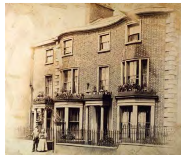
7.7 Town house on Fisher Street (Cumbria Image Bank)
