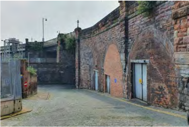
Victoria Viaduct from Bush Brow
