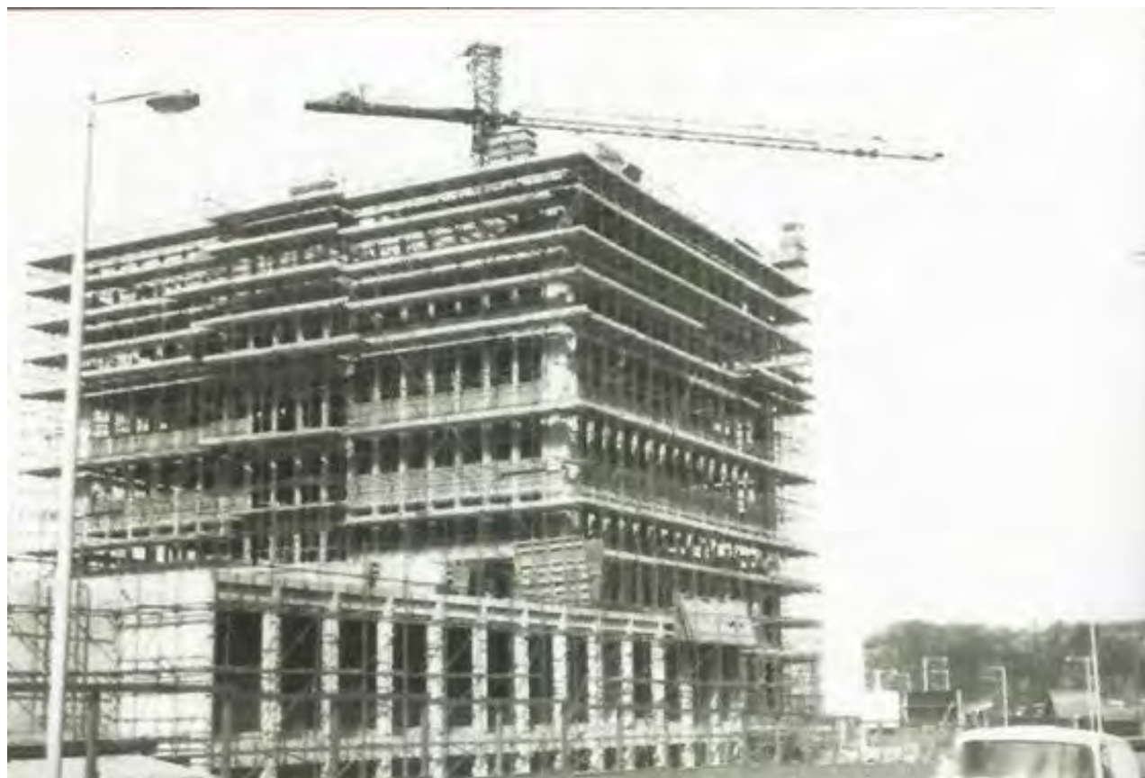
7.21 Civic Centre construction
