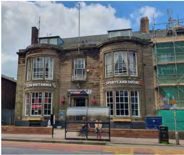
Quality early 19th century town house on the west side of Lowther Street
