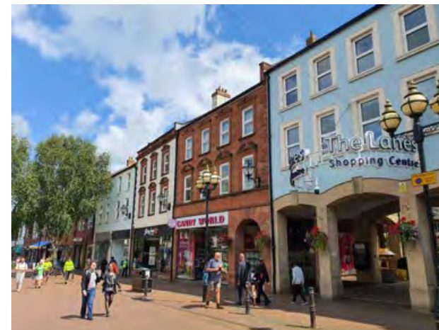
The Lanes Shopping Centre at ground floor level behind modern (some retained) frontages, with apartments to the upper storeys
