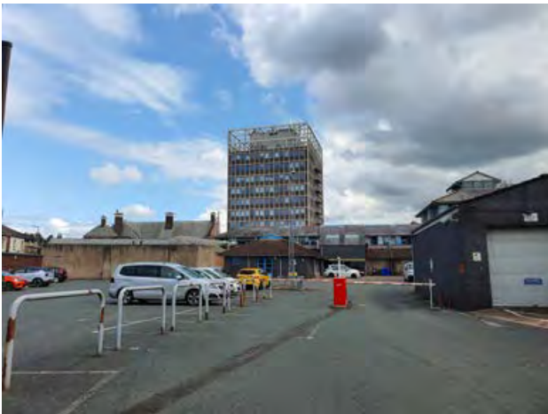
View east across private car park towards the Civic Centre
